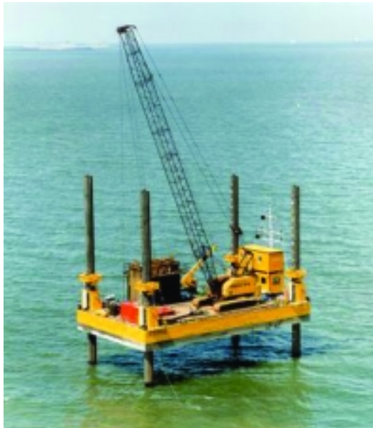
Figure 1: Jack-up barge in position
