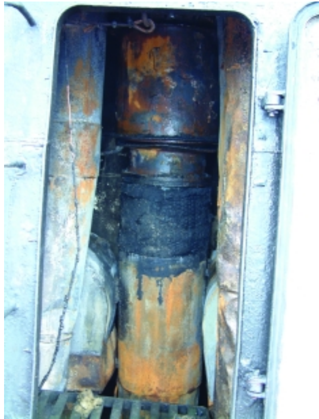
Figure 2: The main engine/silencer arrester – the seat of the second fire
